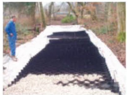
Installation of the CellWeb™ system.
